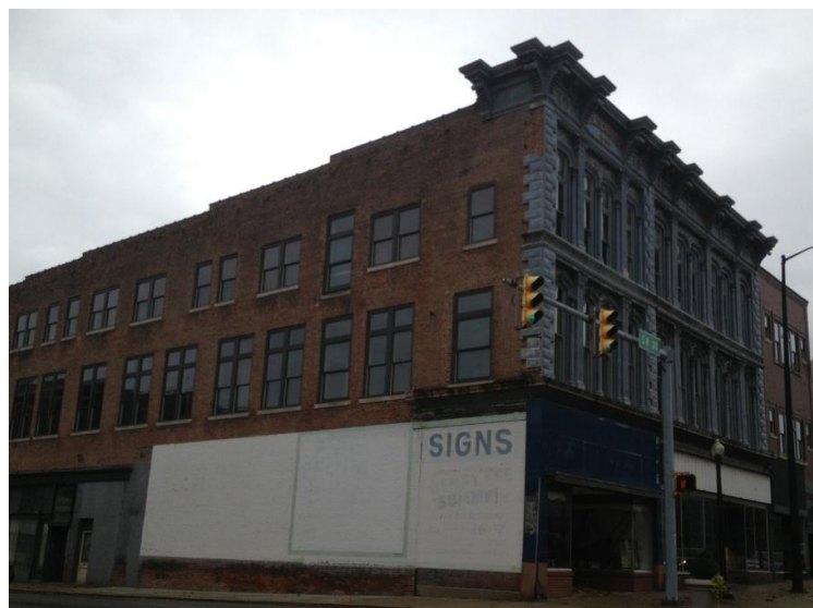
Looking at the site from 14 th and Broad Street.
