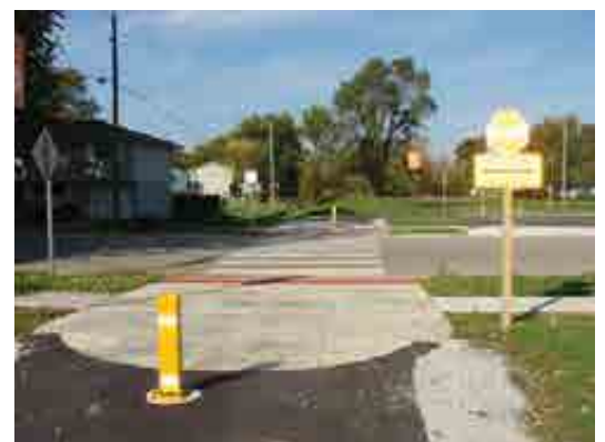
Example of a Concrete Node Entry with Bollard
